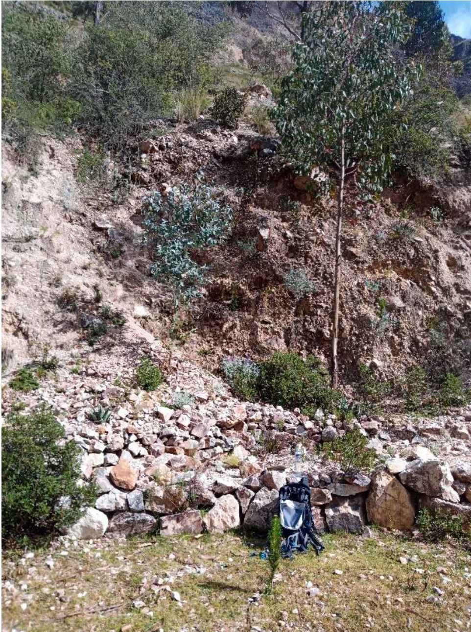
Figure 12-5: Antilla Deposit – Covered Platform for ANT-70-10
